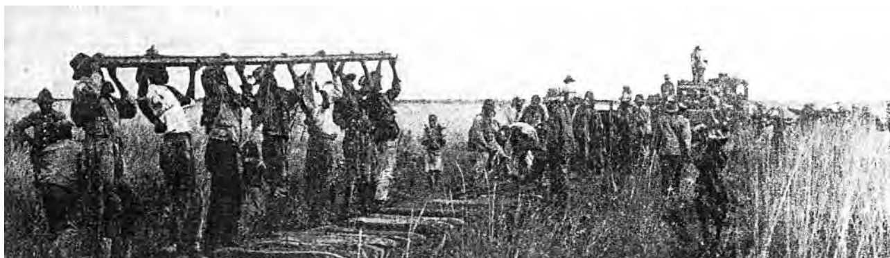
Construction of the Otavi Railway.
